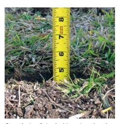
Ensure that installation depth is consistent throughout the installation
